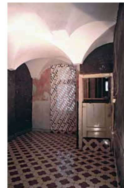
Bar Mysliwska, 1996 Work in progress
